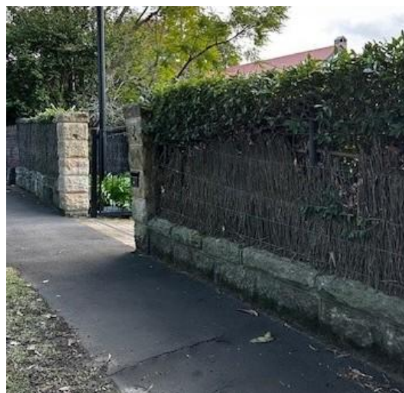
Boundary wall: 32 Ku-ring-gai Ave. Turramurra
